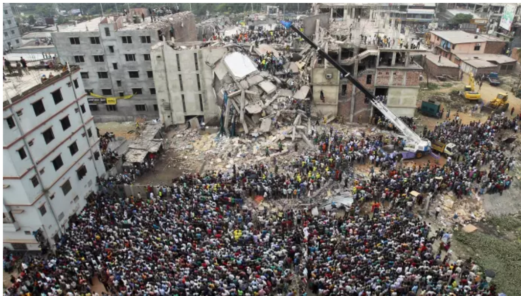
Rana Plaza collapsed on April 24, 2013, killing more than 1,000 people and injuring another 2,000-plus workers © AP
